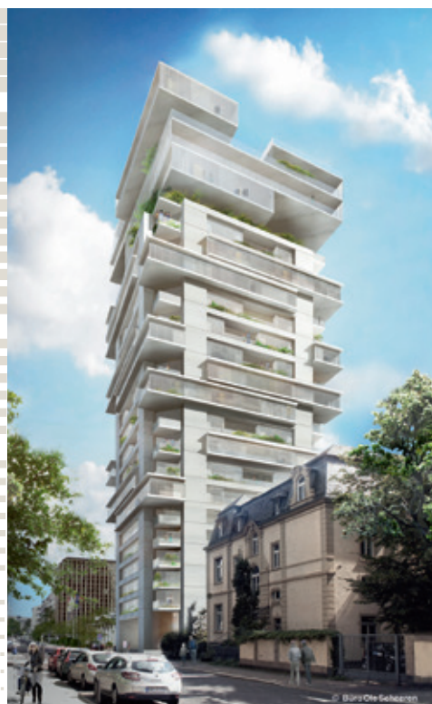
Frankfurt, Riverpark Tower
